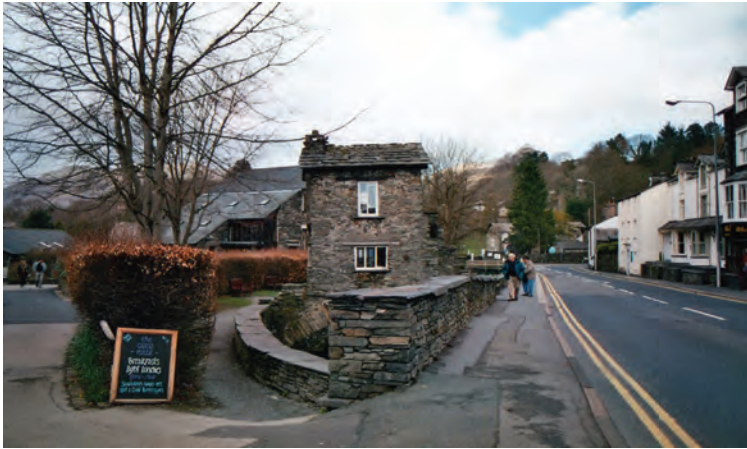
Figure 6: Bridge house, from memory. Ambleside, Cumbria. Author's own (2013).
