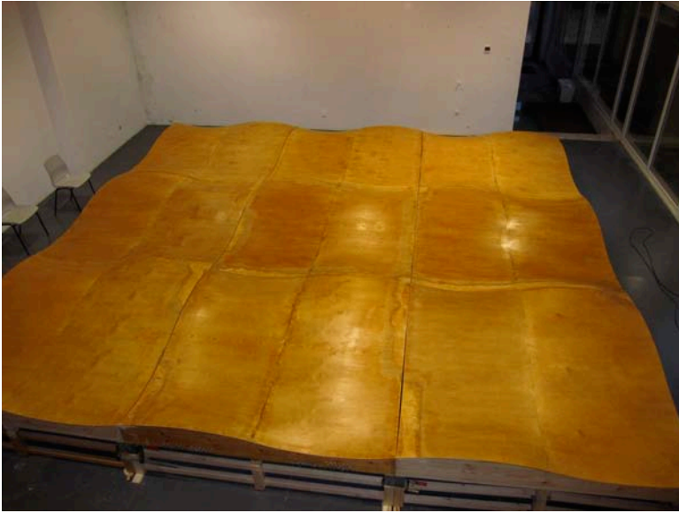
Fig. 8. The final varnish cover enhances the friction sound on the surface. Photo courtesy of Beatriz Cantinho
