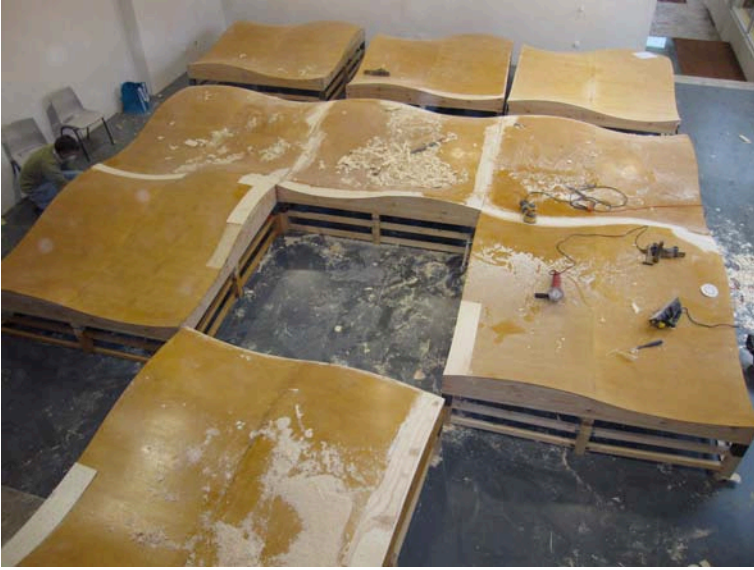
Fig. 6. Aligning the surface. Photo courtesy of Beatriz Cantinho
